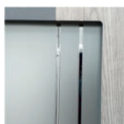
Three-pane glazing with a warm frame system
